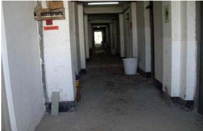
Image: Pearl Tower Dormitory image taken by CLW investigator
